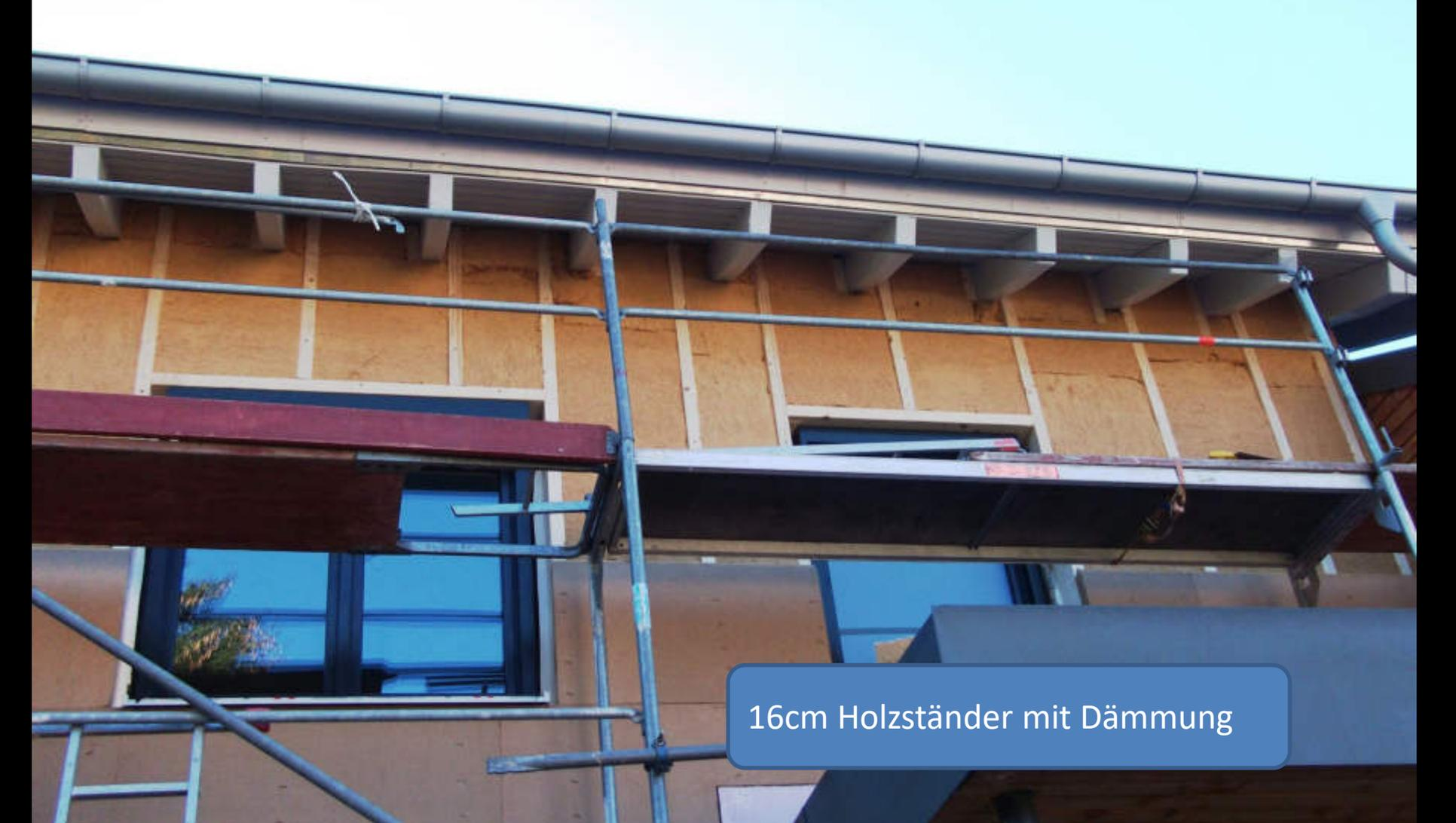
The image shows a close-up of a building's exterior wall during construction. The wall is framed with light-colored wooden studs and filled with a light brown insulation material. A metal scaffolding structure is visible in the foreground, with a red horizontal beam. A dark window frame is partially visible. A grey downspout runs along the top edge of the wall. A blue text box is overlaid at the bottom right.
